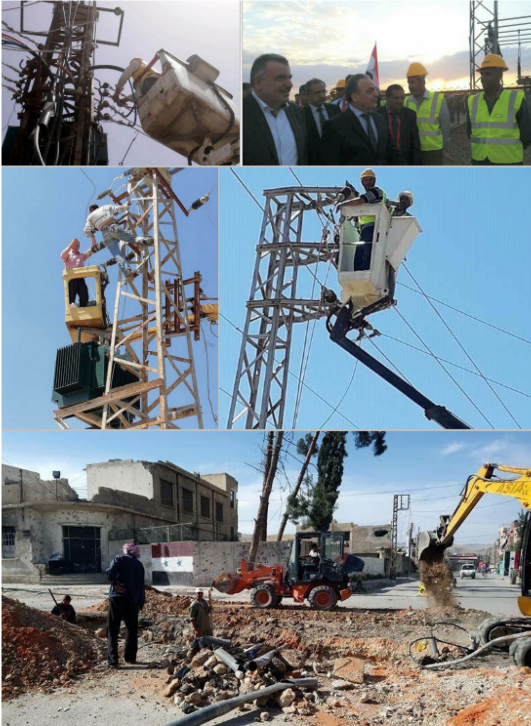
The rebuilding electricity infrastructure in Douma and Nabaa al-Sakhar
