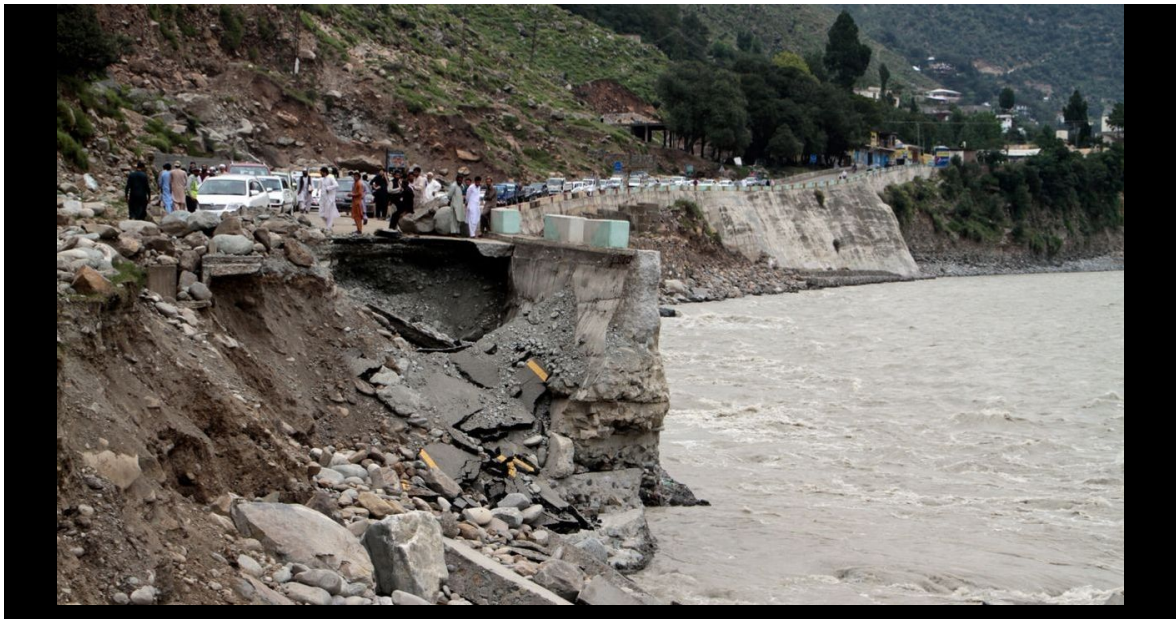
Passengers wait by a damaged road next to floodwaters, in Bahrain, Pakistan, Tuesday, Aug. 30, 2022. [AP Photo/Naveed Ali]
