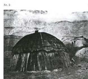
Fig. 5. "Chapar" completely covered with straw from the Hazara between Dikhel and Puli-Schamir. The frame consists of curved sticks and there is no central pole. This type is also found with mats and felt cover. (Phot. by Peter Baumeister, November 1953).
