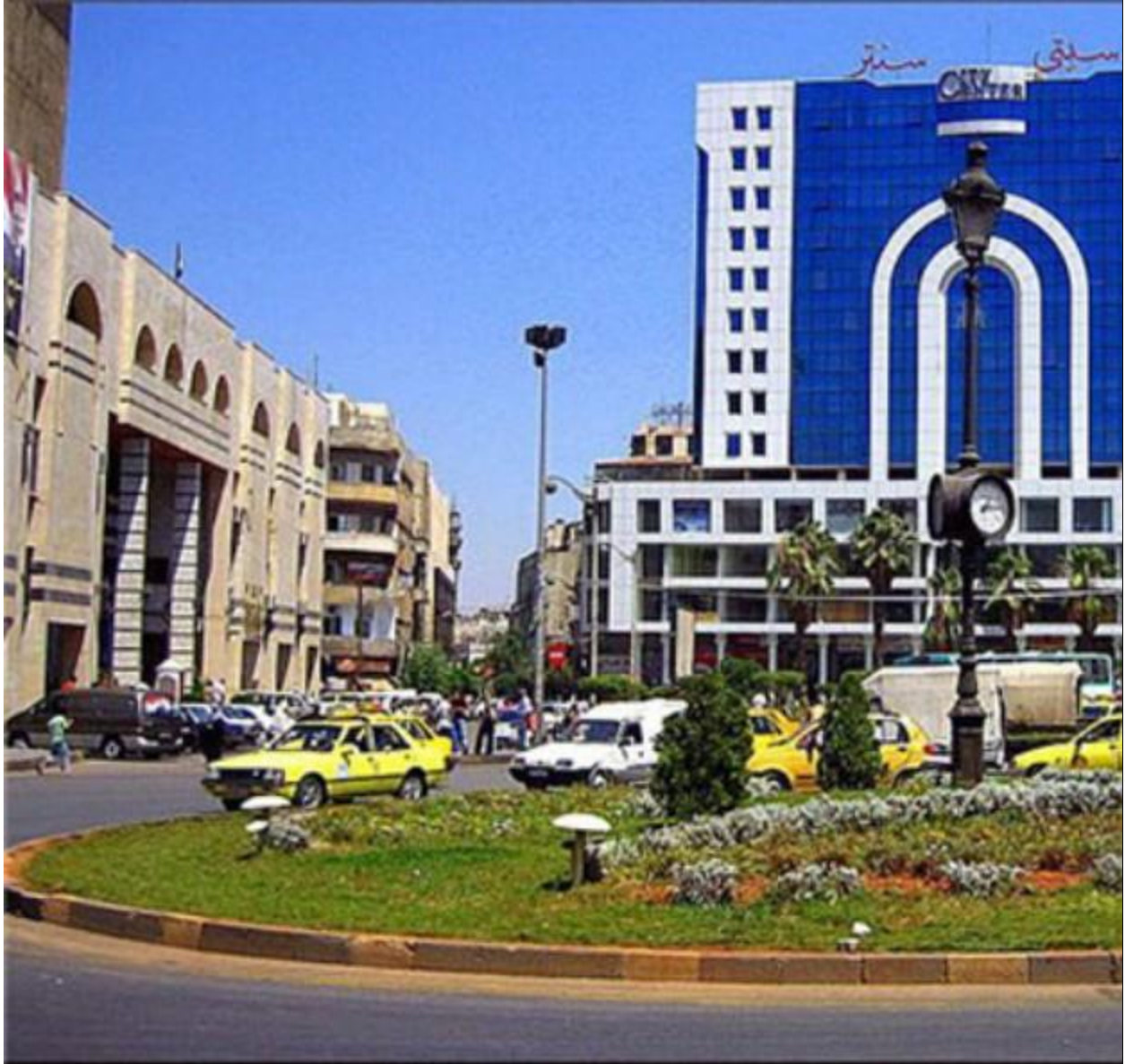
Homs city centre mall, located in the commercial district, has been heavily damaged by the fighting between regime forces and rebels.
